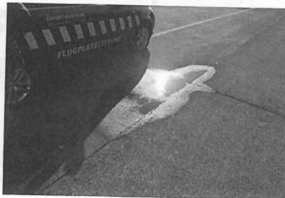
Diagonalstrasse Ost / Rwy Charlie
