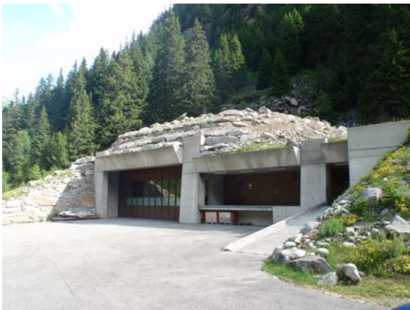
Service building (storage facility and workshop for vehicles)
