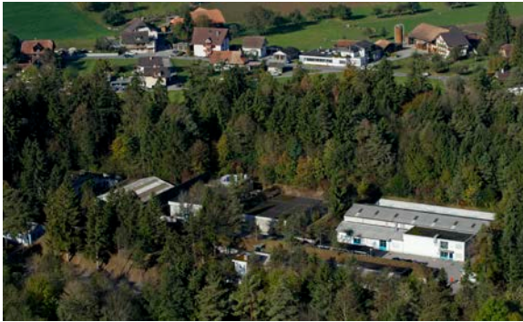
Overall view of Thierachern Facility
